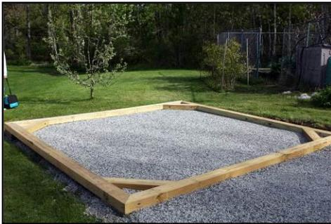
The ground that the Freedom Greenhouse sits on does not have to be level, but the base for the greenhouse does need to be both square and level. The other requirement of the base is that it is anchored against moving. Strong winds or a bump from a lawn tractor can move a greenhouse if not firmly anchored.
