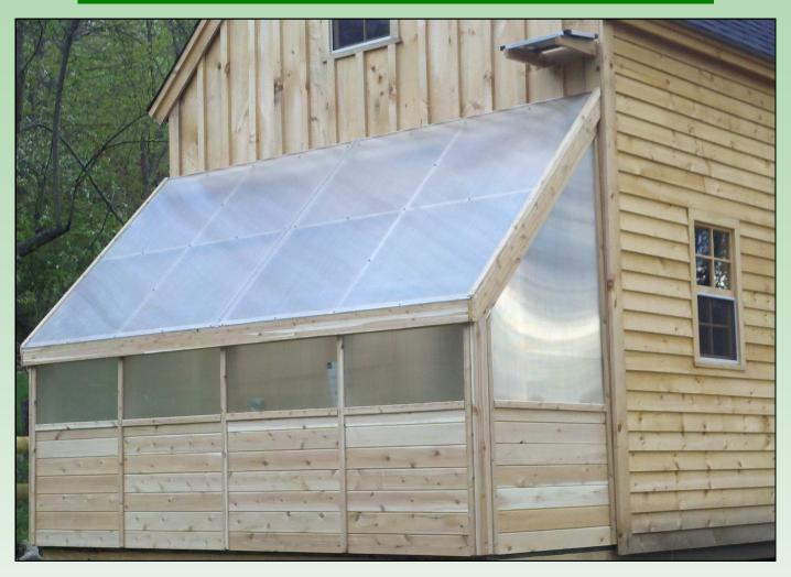
Freedom Greenhouse Lean-to structures can be made to attach to a variety of existing structures. Custom made and available in sizes from 4' deep x 8' long up to 12' deep x unlimited lengths. As with all Freedom Greenhouse structures they feature natural convective ventilation and can be solar panel/battery powered or 120v charger/battery powered. Multiple configurations and door options on all sizes. NEW options include glass sidewalls and gable ends for all greenhouses.
